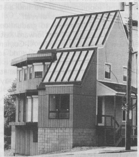
The Solar House
