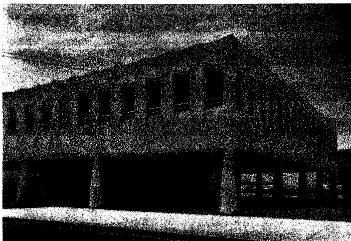
Catechetical Center, Christ The King Church, Ambridge, Pennsylvania Architect: Belli & Belli Chicago, Ill. Contractor: Hammerberg Const. Co. Pittsburgh, Pa.
