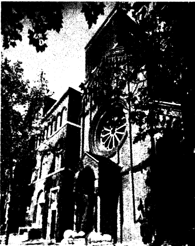
Facade of the Fleisher Art Memorial (former Church of the Evangelists) today.
